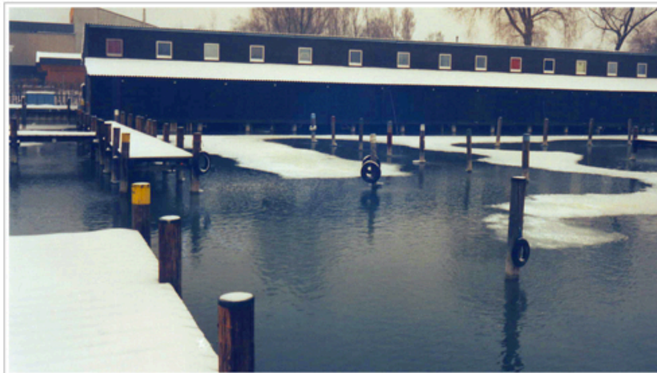
Ice Prevention Plant at -20°
