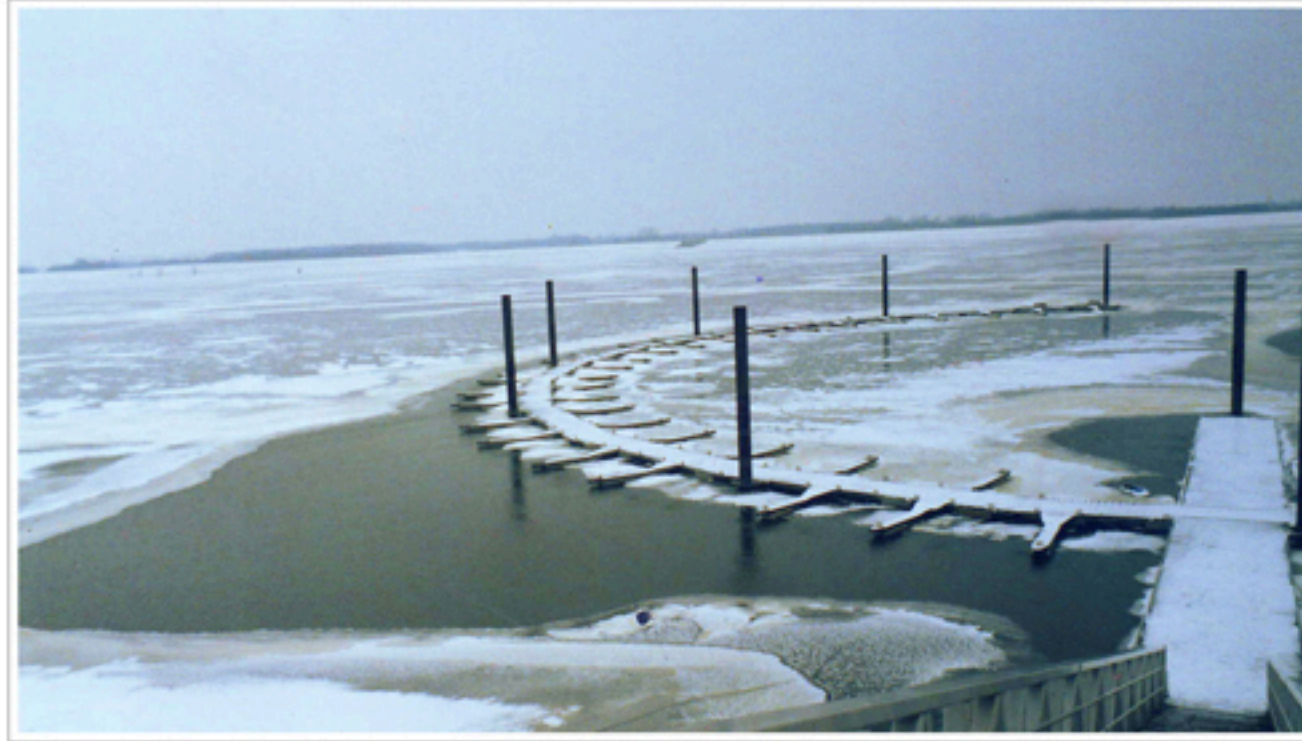
Ice Prevention Plant
