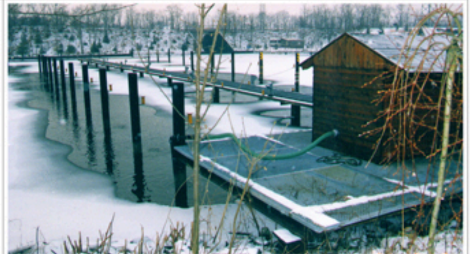
Ice Prevention Plant, Braunschweig
