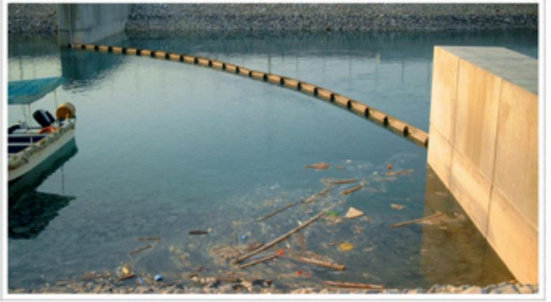
elements. These adjust to the respective water level by means of slide rails. If the water level is rising, the passage beneath the barrier increases. Water can flow out at an even, low speed. Oil or floating debris is held back by the floating body on the surface.
