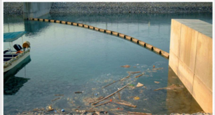
elements. These adjust to the respective water level by means of slide rails. If the water level is rising, the passage beneath the barrier increases. Water can flow out at an even, low speed. Oil or floating debris is held back by the floating body on the surface.
